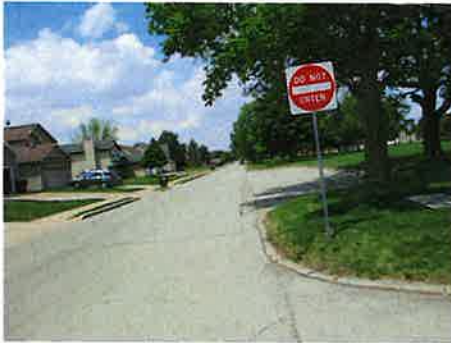
Diversatech Drive (south) looking west.
