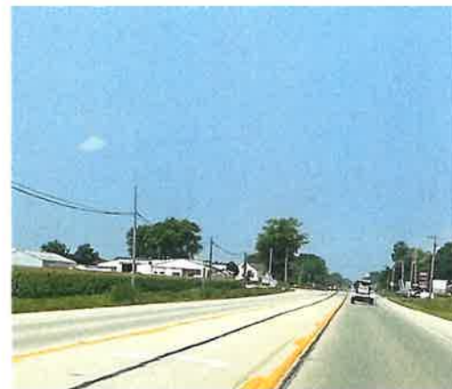
IL Rt. 17 looking west.
