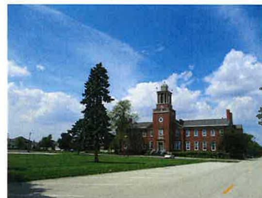
Subject Site Looking west.
