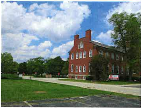
Subject site looking north.
